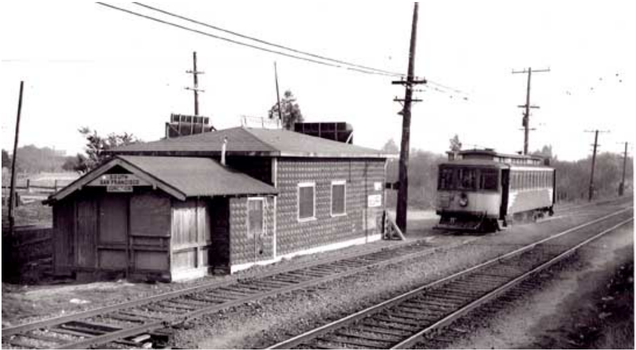
Historic Photo 2 Leipsic Station in South San Francisco, undated
